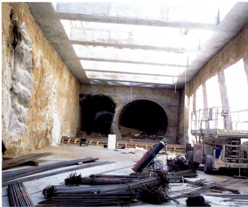
TBM removal point outside Cuatro Vientos station.
