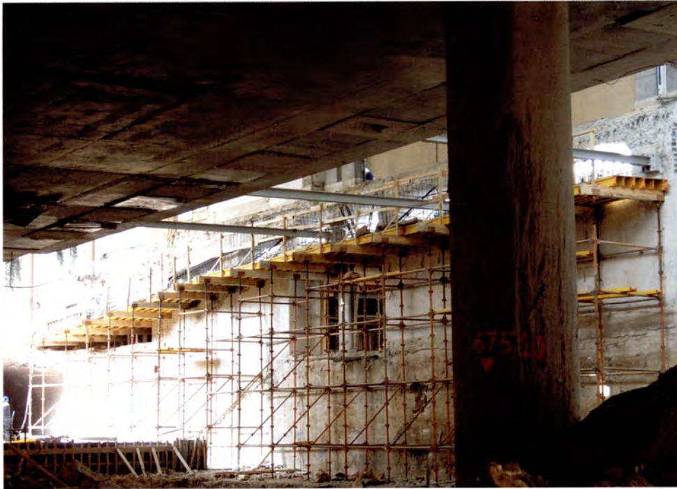
Voids for the passage of support and tying beams at Nuevos Ministerios arcade.
