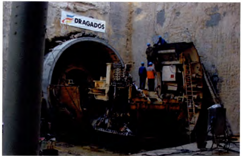
Final dismantling of Lovat TBM.
