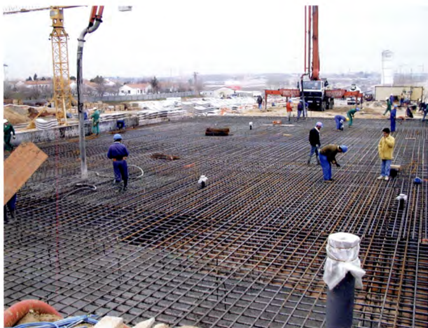
Laying the concourse roof at Colonia Jardín.
