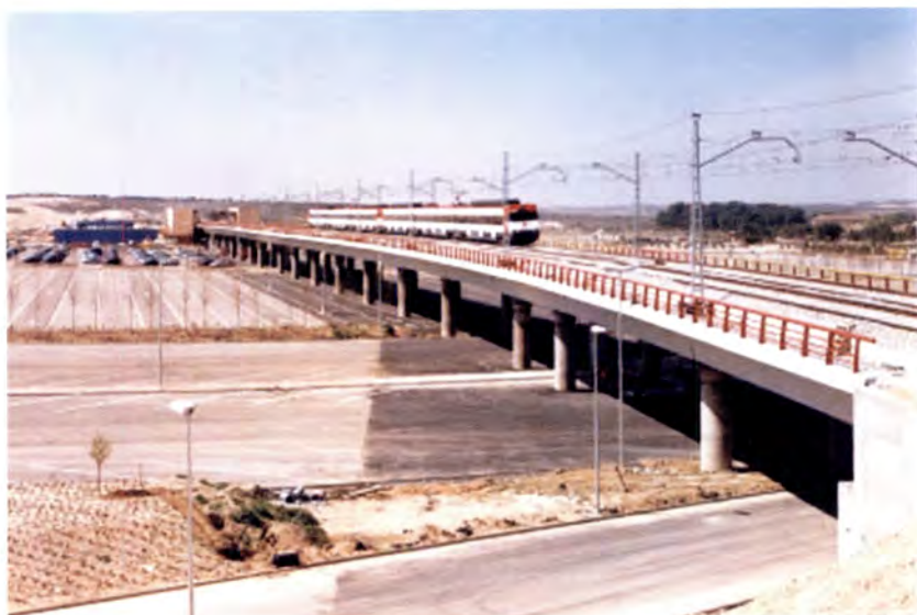
Theme park viaduct.
