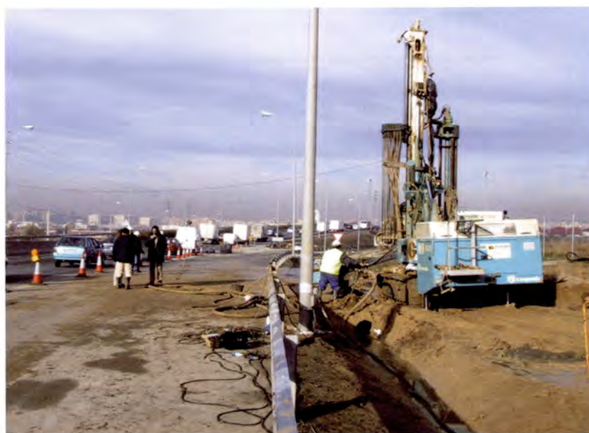
Cement injection on highway M-406.
