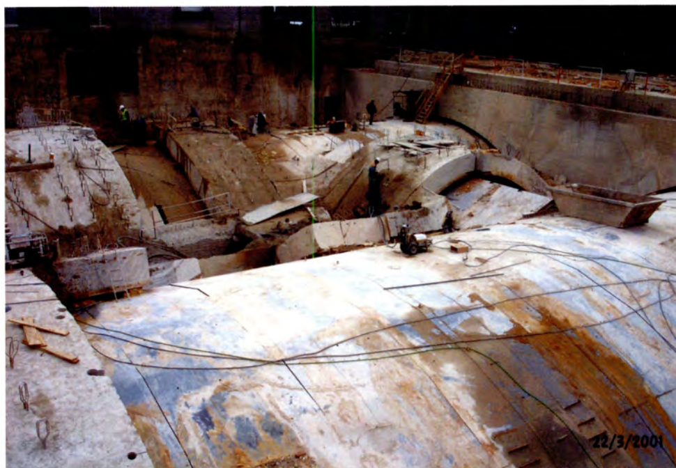
Transverse cuts for the introduction of steel framework over RENFE line tunnels.
