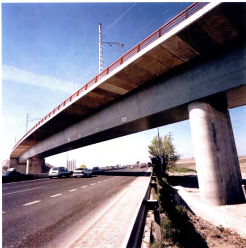
Viaduct over the N-IV highway.
