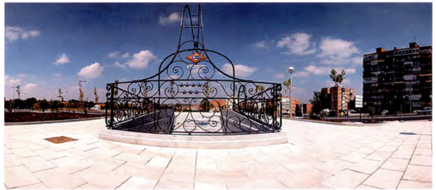
Patio station entrance.
