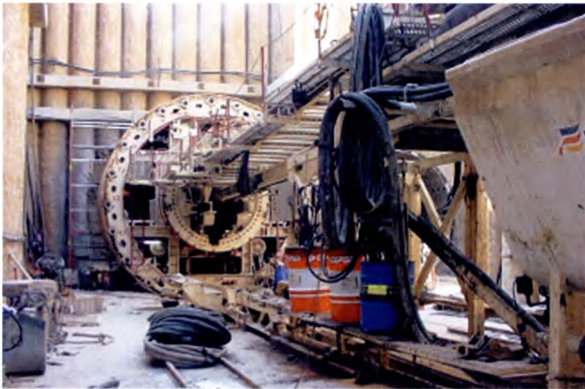
TBM assembly at telescope 2.
