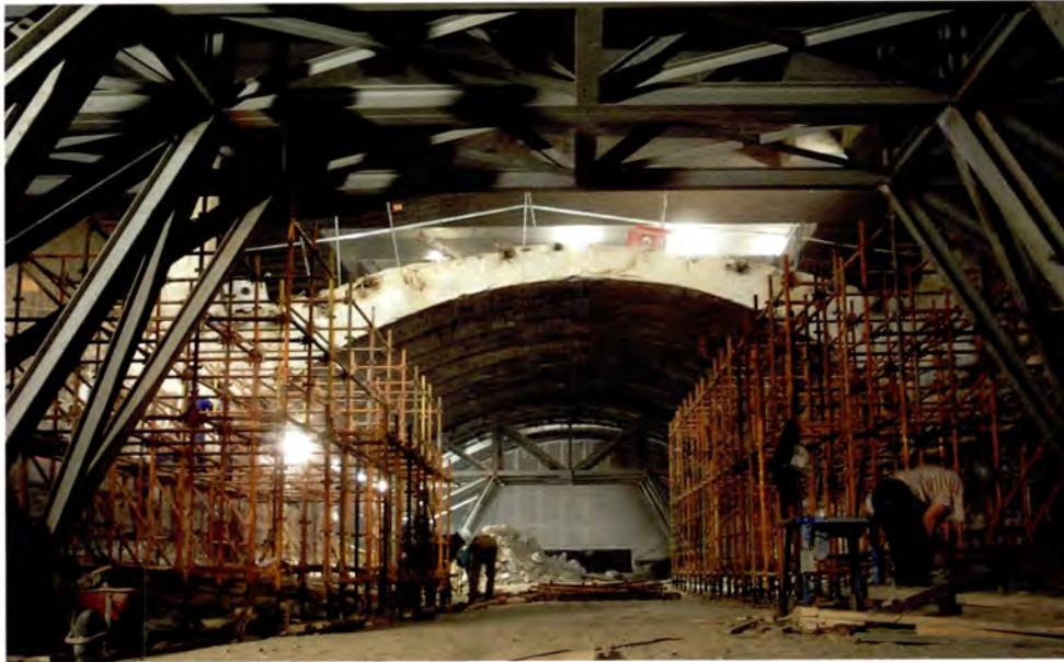
Cutting line 9 roof vault at Colombia station.
