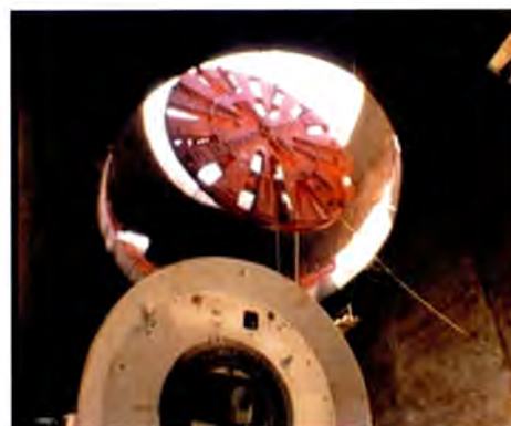
Lowering the cutterhead of the Herrenknecht TBM.
