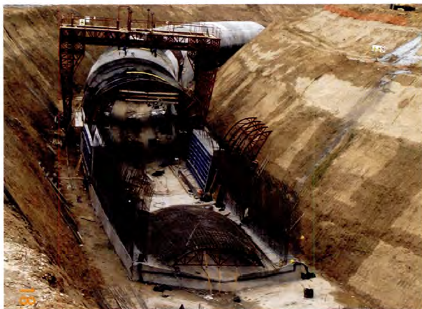
Open cut tunnel under construction.
