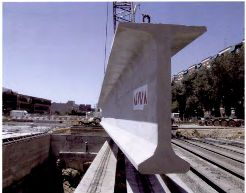
Placing the roof beams at a station.
