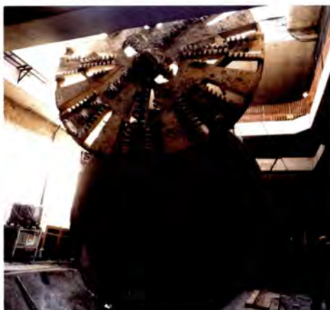
Removing TBM cutterhead through G2 shaft.
