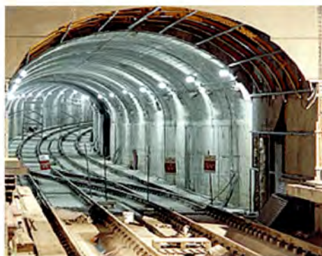
Traditional tunnel from Loranca station.
