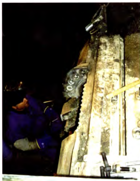
Repairing TBM cutting head at PK2 +589 shaft.
