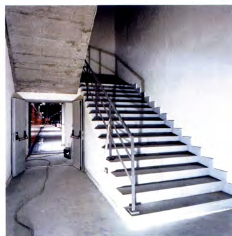
Emergency exit stairway.
