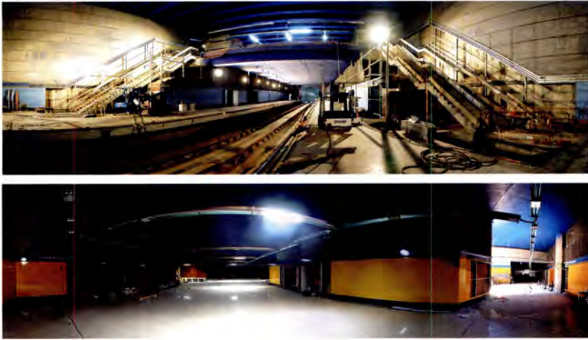
Loranca and Fuenlabrada Hospital stations nearing completion.
