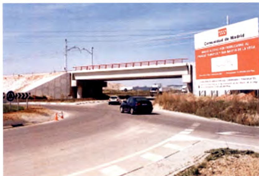
Overpass at the M-301 road.
