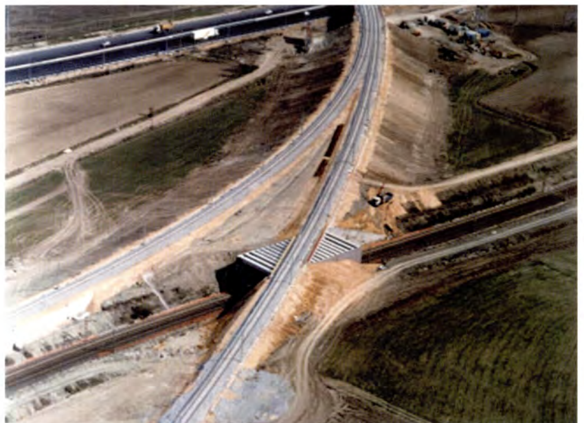
Flyover with embankments.
