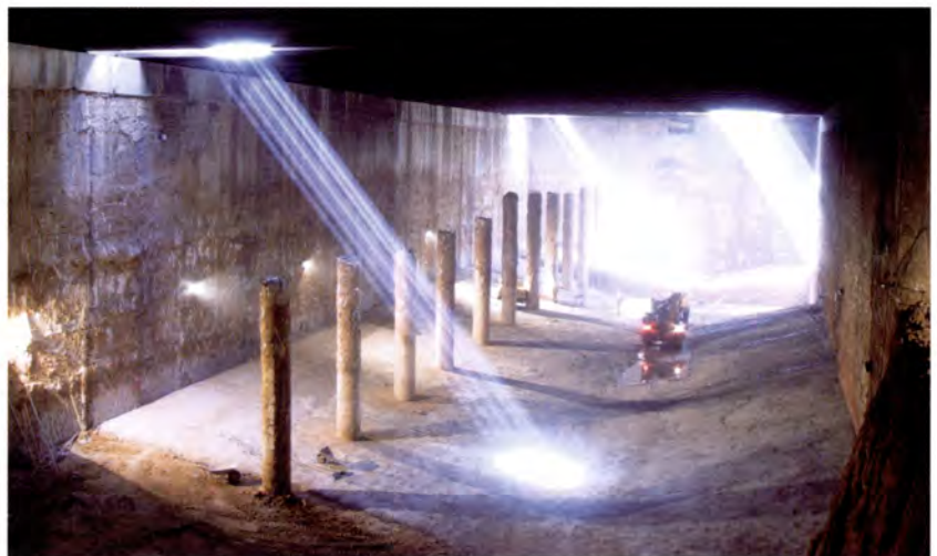
Beamed roof and invert slab with mezzanine support pillars at Alcorcón 3 station.
