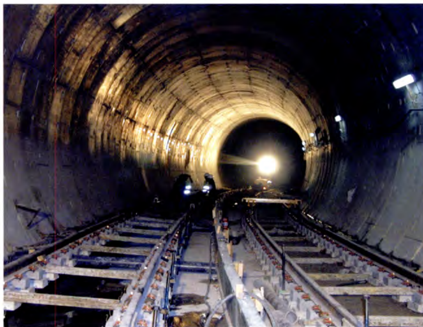
Tracklaying in the completed TBM tunnel.
