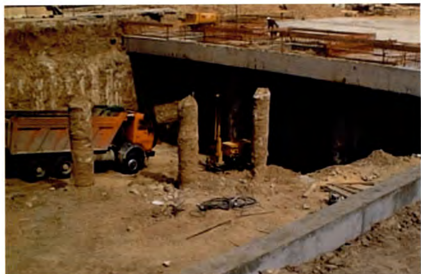
Excavation beneath the roof slab of Joaquín Vilumbrales station.
