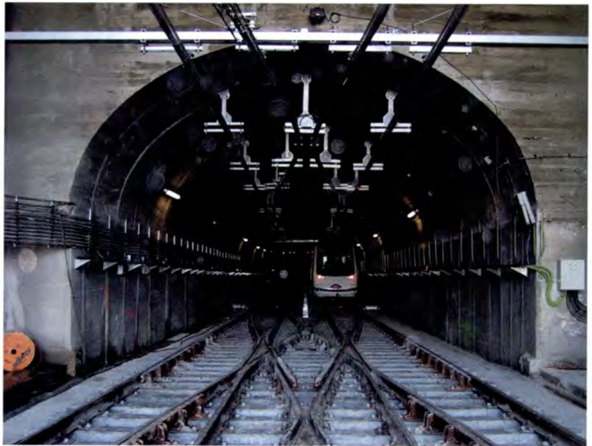
Access tunnel portal.
