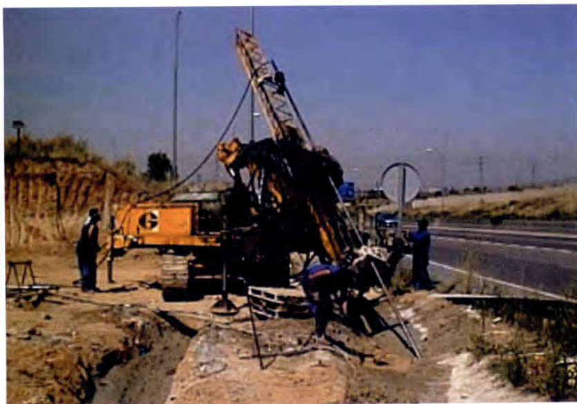
Jet grouting columns alongside M-40 motorway.
