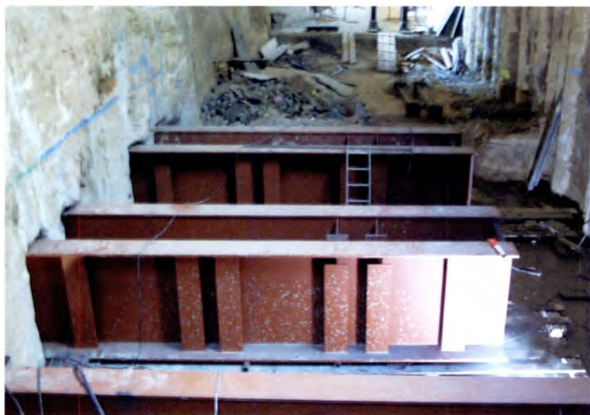
Supporting beams for the carpark slab.
