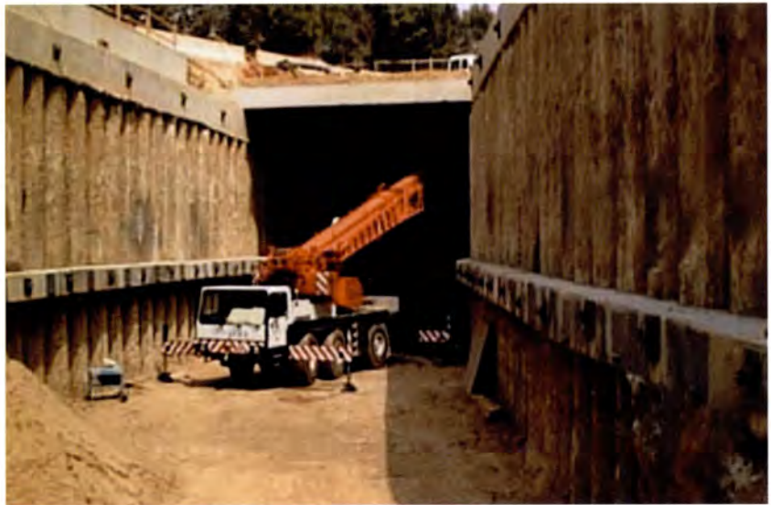
Telescope 1 with provisional anchorages.
