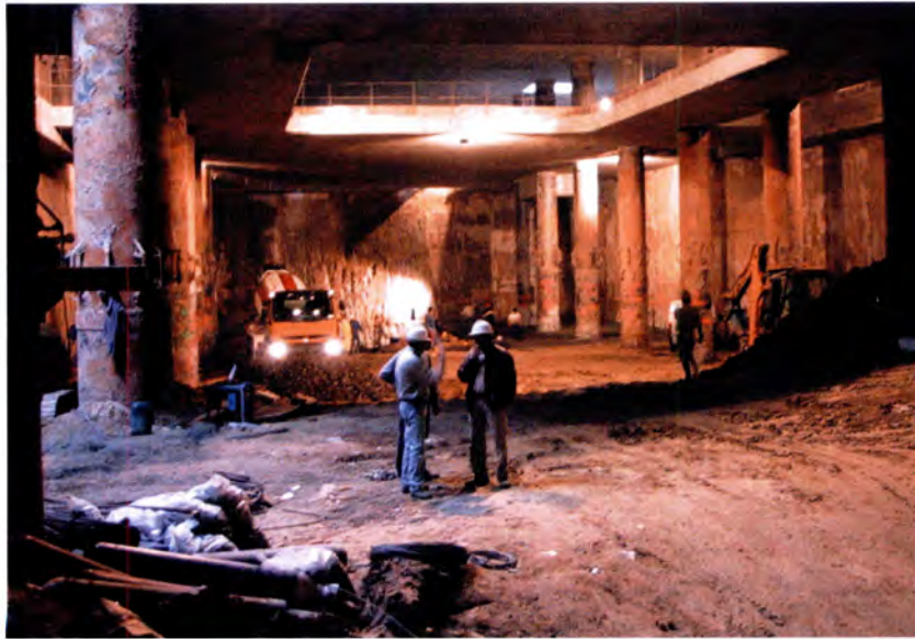
Excavation of Casa del Reloj station prior to TBM arrival.
