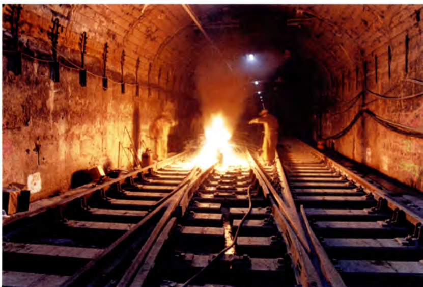
Installing track assembly.
