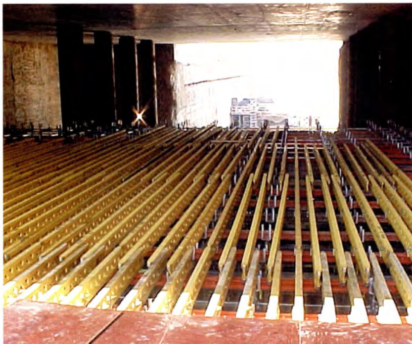
Formwork for concrete mezzanine floor at Colonia Jardín.
