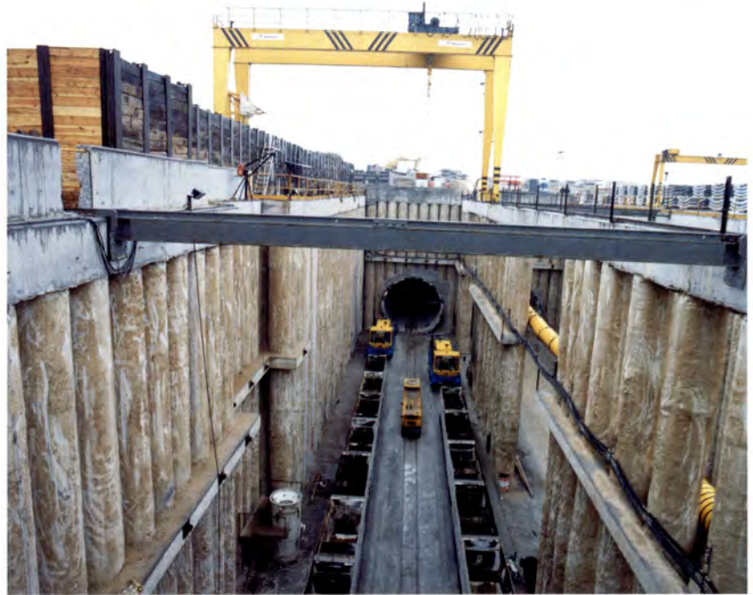
TBM launch chamber at Mimbreras.
