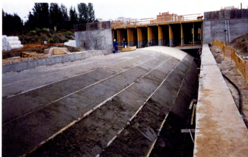
Arched station roof under construction.
