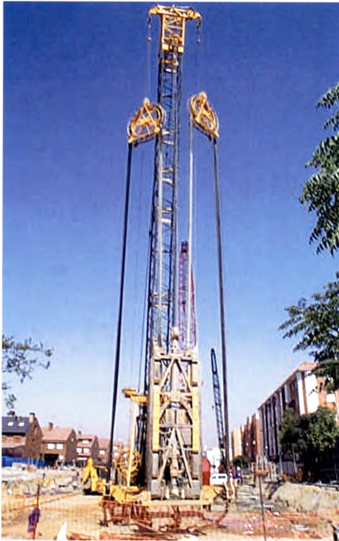
Hydrocutter at Espartales station.
