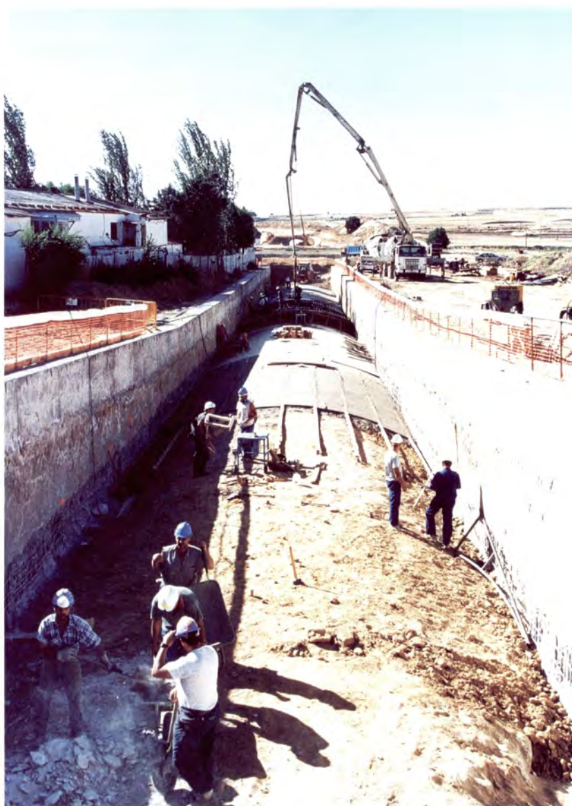
Roof concreting between screen walls.
