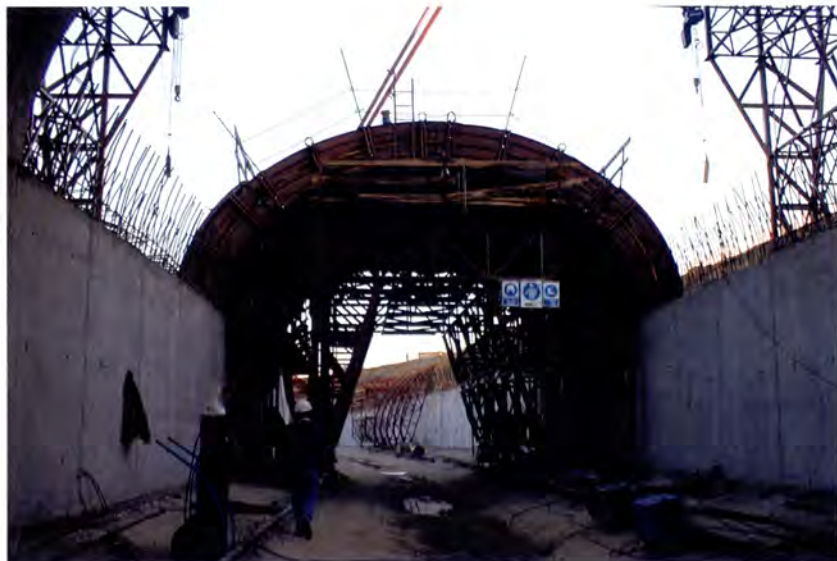
Travelling roof formworks in open cut.
