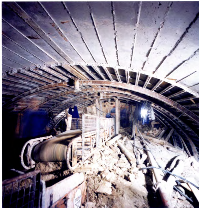
Spoil conveyor from top heading face.
