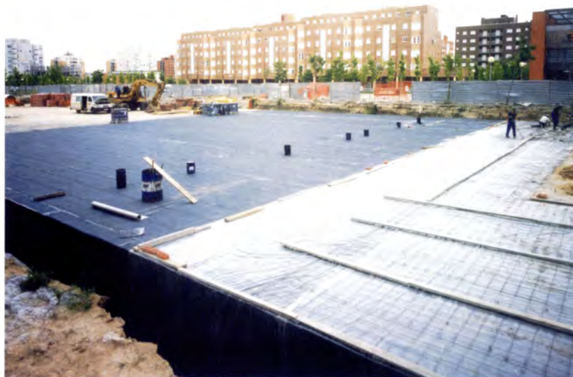
Concrete cover of Fuenlabrada 1 station.
