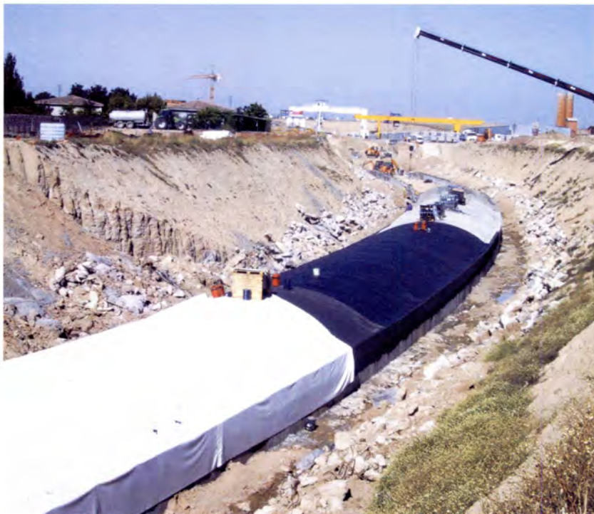
Applying the waterproofing layer to the external roof of the cut and cover tunnel.
