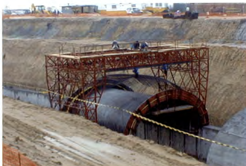
Gantry placing prefabricated roof reinforcement.
