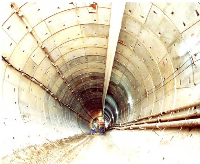
Cleaning up in completed TBM tunnel.
