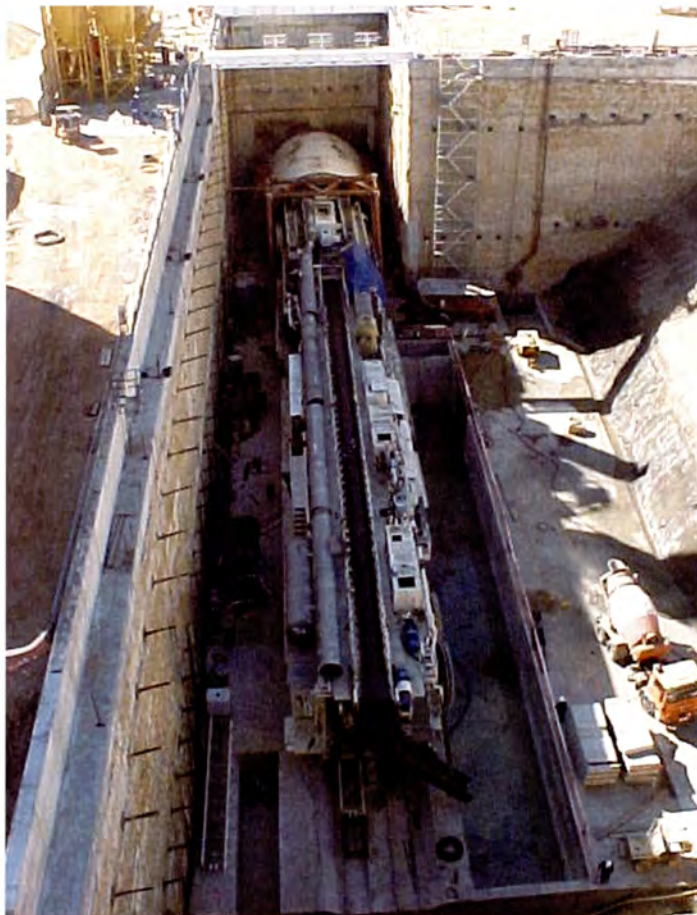
Adelantada ready for launch using the reaction frame.
