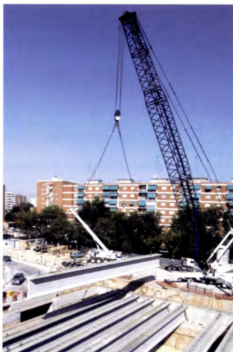
Crane positions the final beams to close a station roof.
