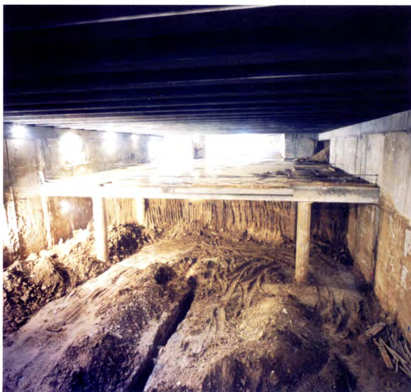
Mezzanine floor at Fuenlabrada 1 station.
