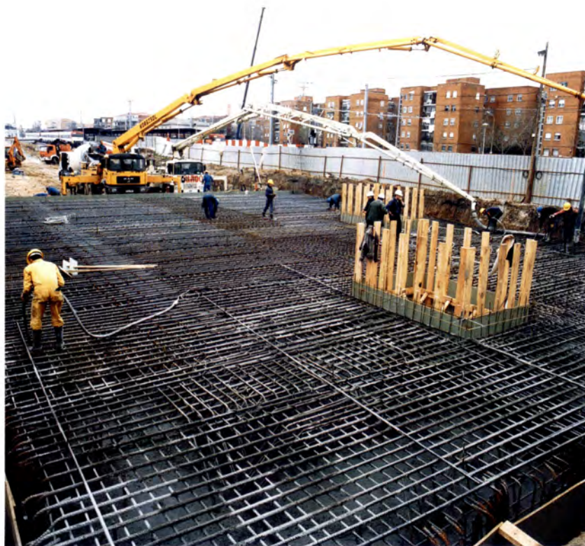
Pouring the concrete roof of a station box.
