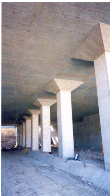
View through the box jacked section.
