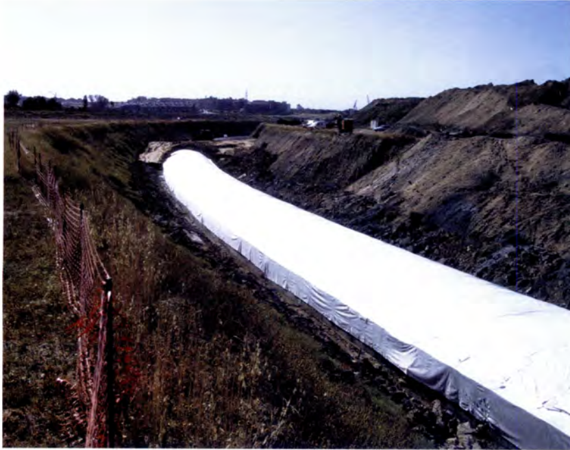
Curved section of cut and cover tunnel near Leganés.
