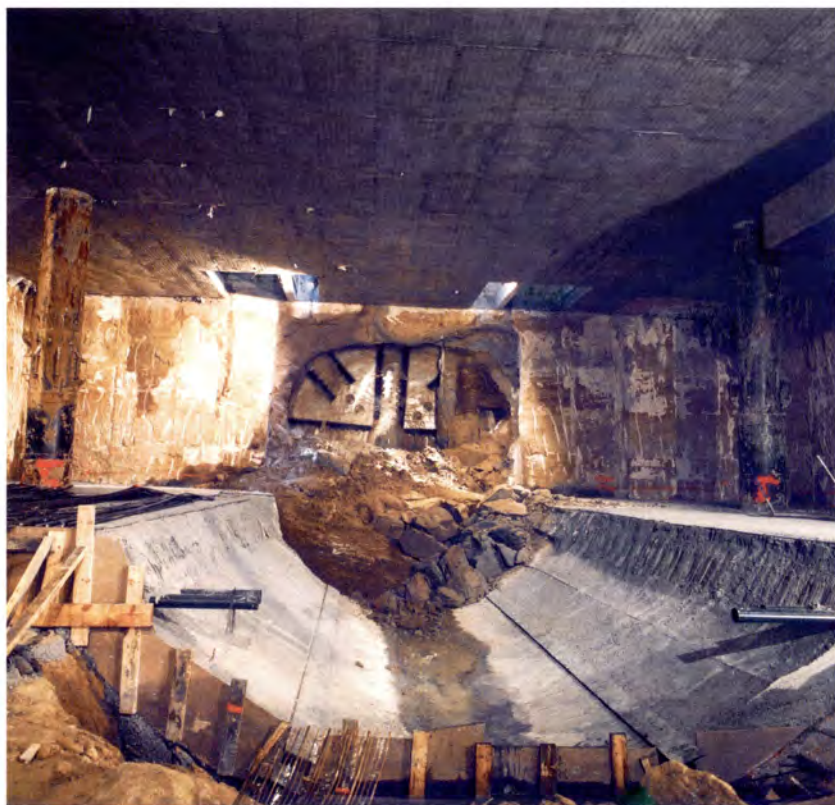
TBM breakthrough into a half-constructed station.
