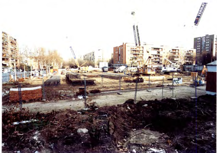
Screen wall installation at Móstoles 4.
