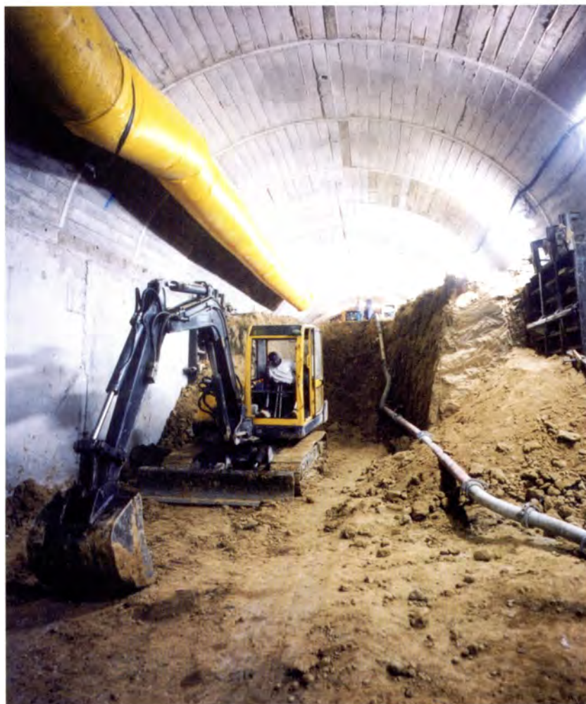
Excavating sidewalls of traditional tunnel.
