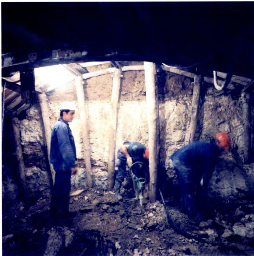
Traditional Madrid method of excavation.
