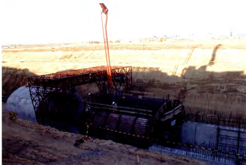
Pouring concrete into the formworks.
