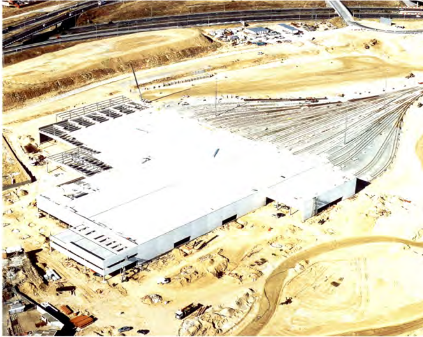
Depot main building will house 30 tracks.
