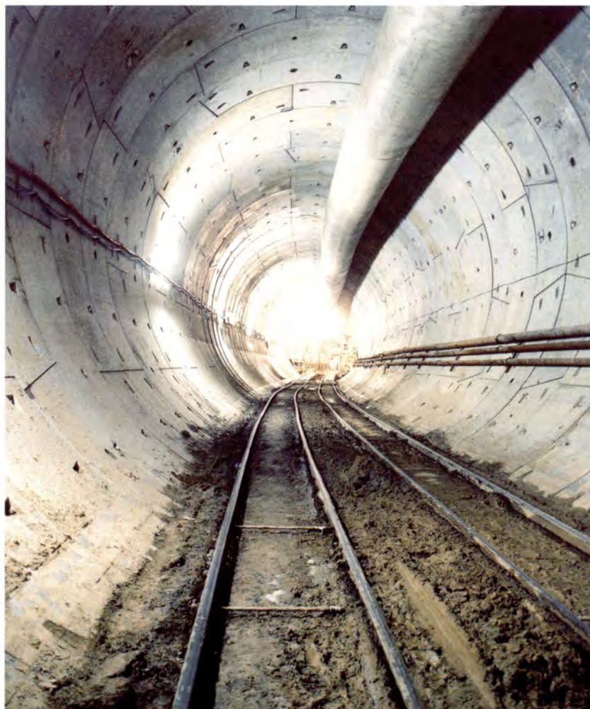
Stretch of finished TBM tunnel.
