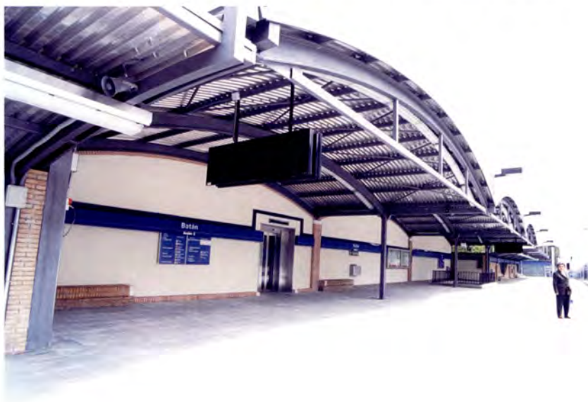
Covered platform area at Batán station.
