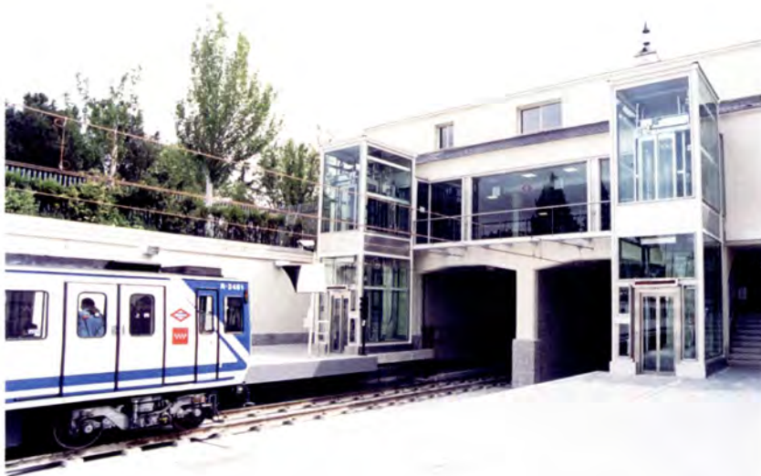
Completion of Lago station and tunnel widening.
