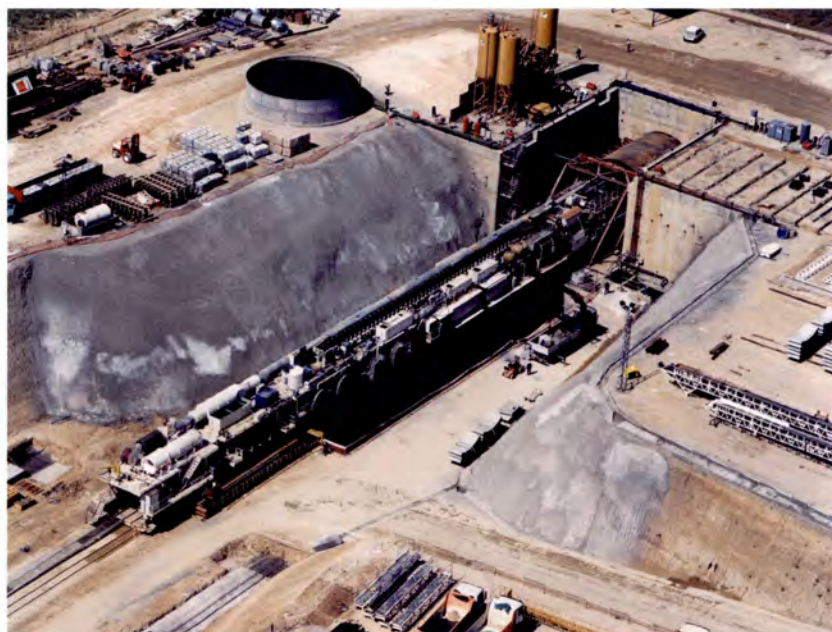
La Adelanta TBM installation at Móstoles 5 station.
