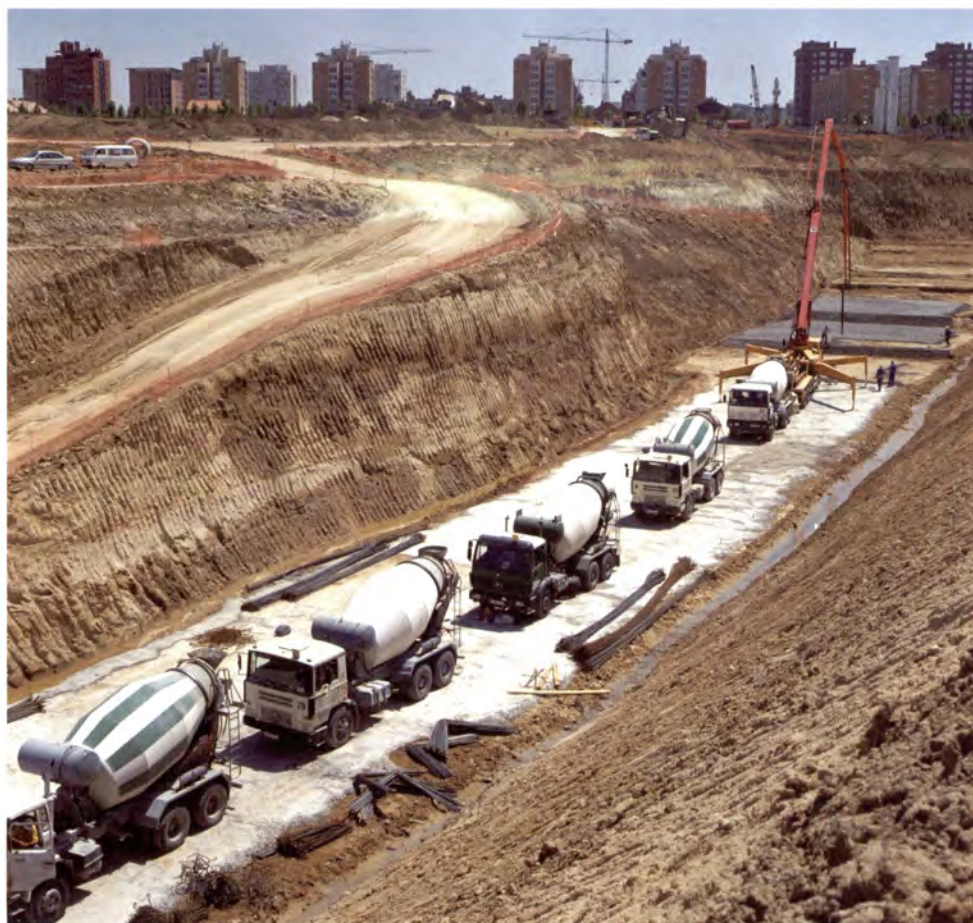
Casting the floor slab of the three-track telescope section.
