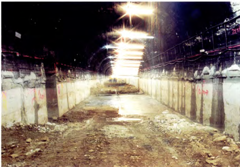
Underpinning a stretch of tunnel.
