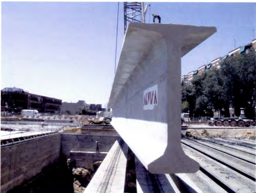
Placing the roof beams at a station.
