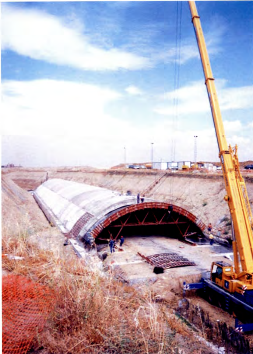
Construction of future station roof.
