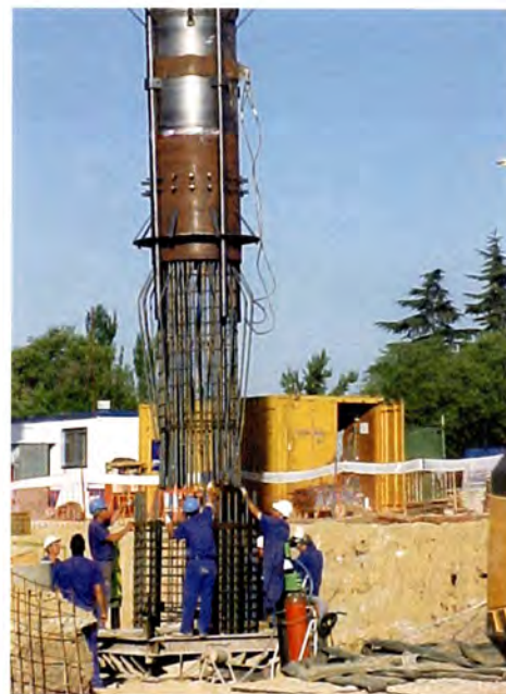
Installing a station roof support pillar.
