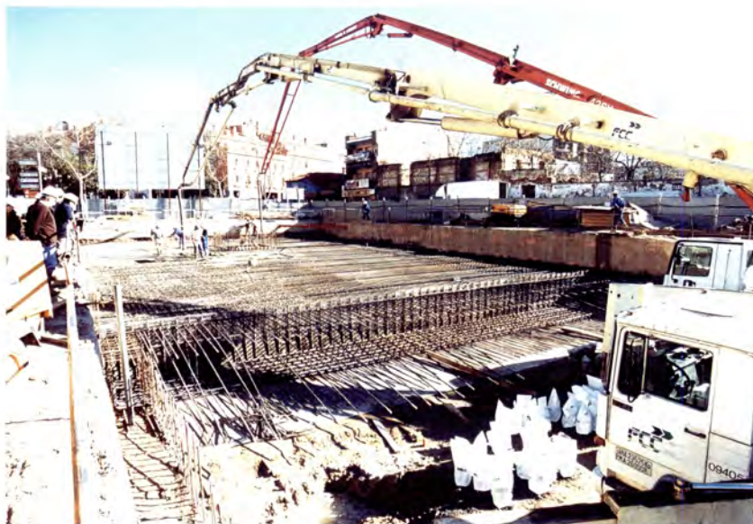
Roof slab concreting at Móstoles 3.
