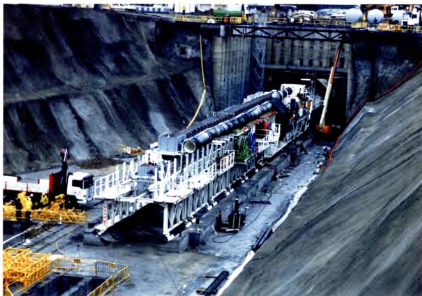
Launch pit for Herrenknecht EPB at El Bercial.
