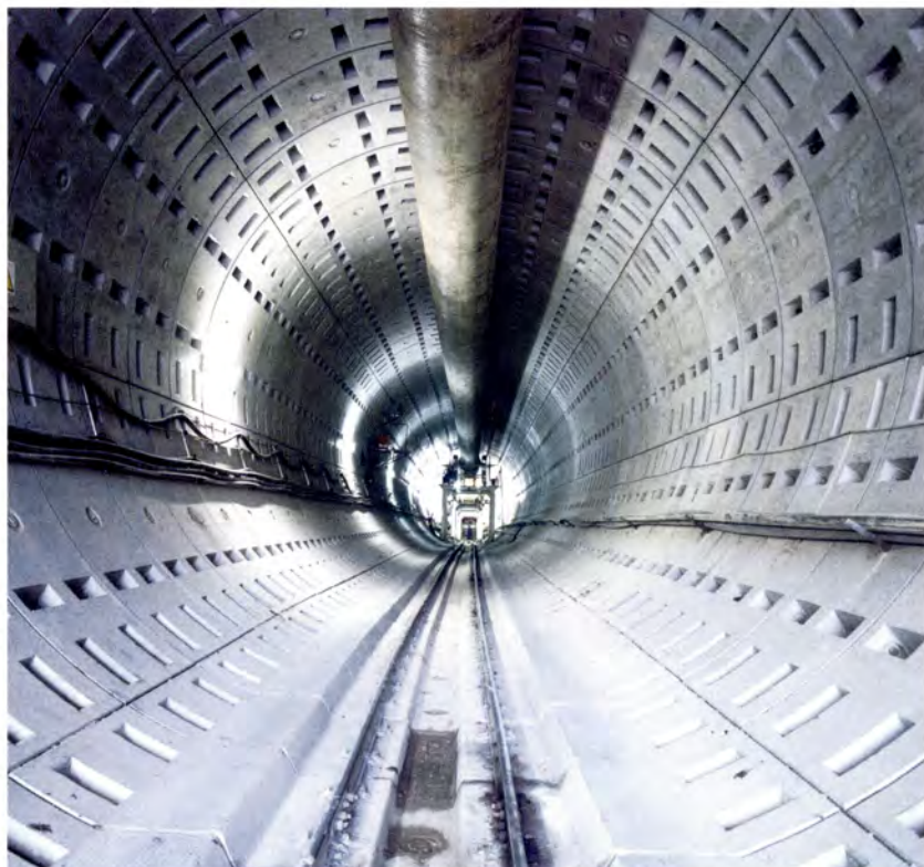
Section of completed tunnel shows the Zephir tracks.
