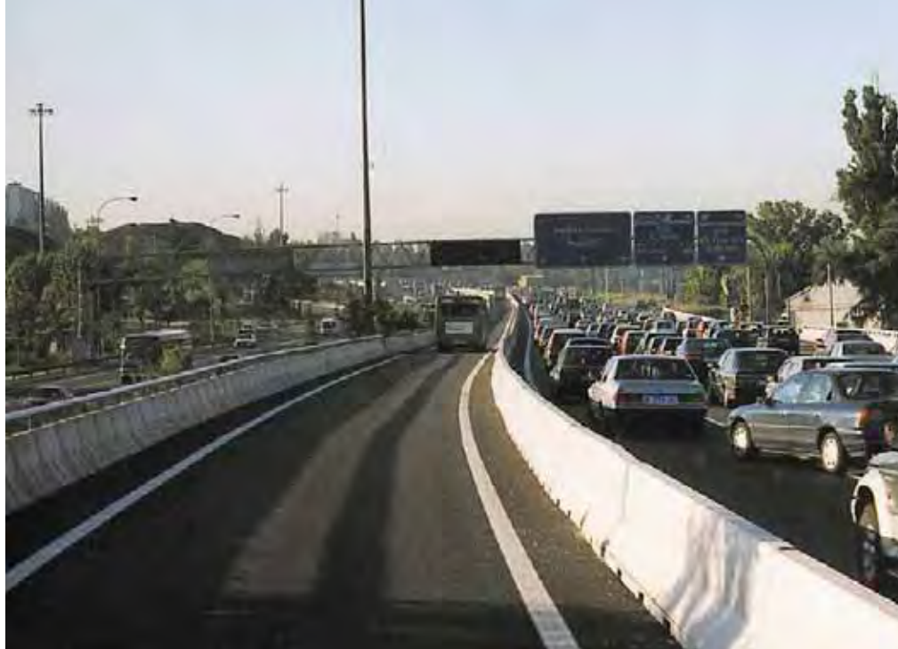
Carril Bus-Vao de la A6 / The Bus-HOV lane on the A6 road
