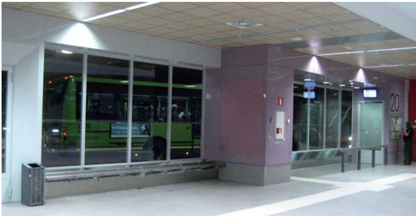
Mampara perimetral / Perimeter screen wall
