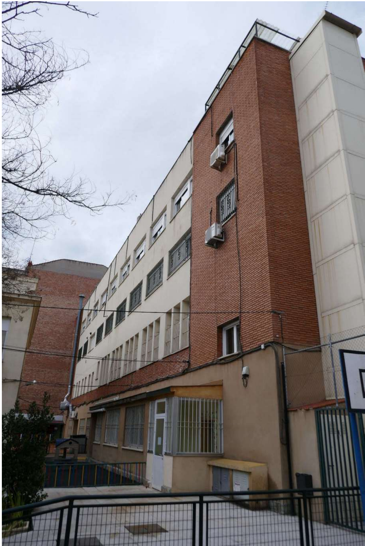
FACHADA A PATIO INTERIOR
