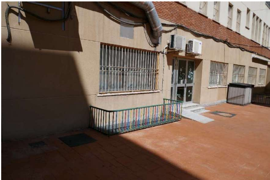
FACHADA A PATIO INTERIOR
