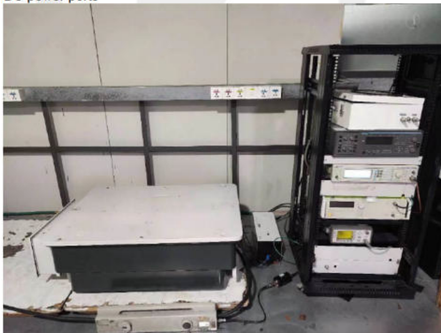
DC power ports
